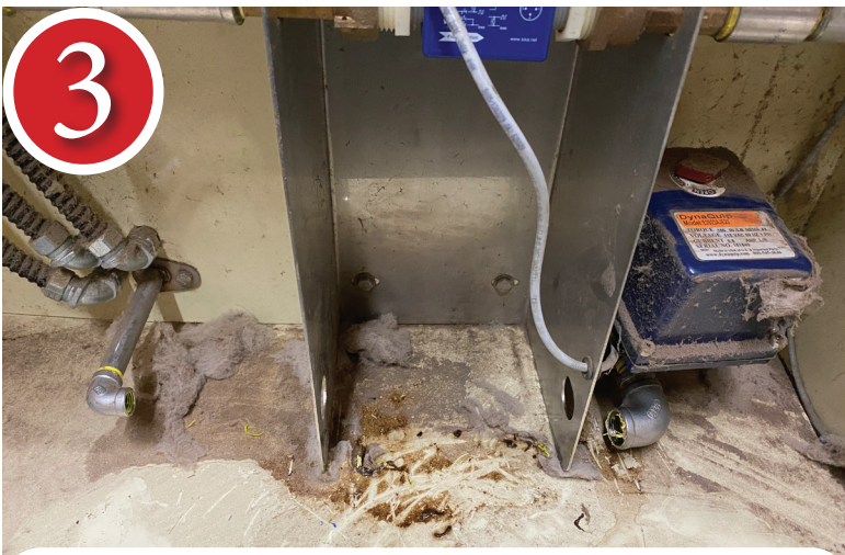
Remove pipe back to elbows
