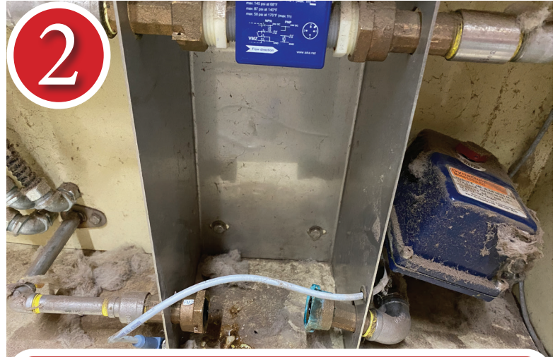
Remove old water meter
